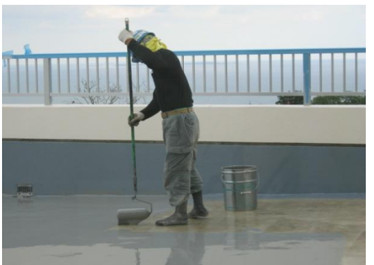
7. Application to waterproof treatment
