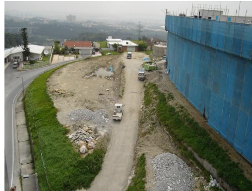
Nov. 2005 preparation of the construction
