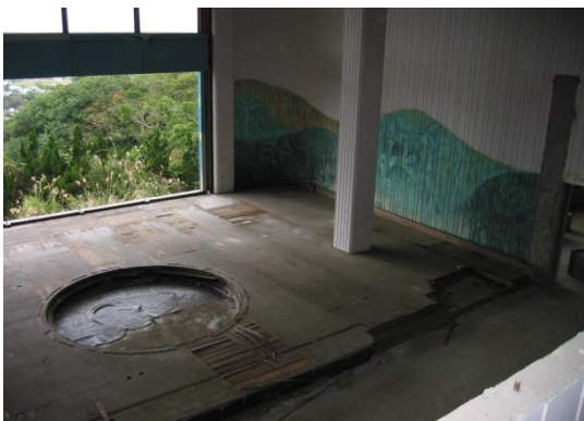
Bar lounge on the first basesment level
