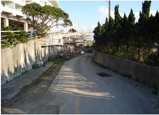
A carry-in entrance
