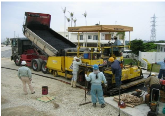
5. Application to asphalt
