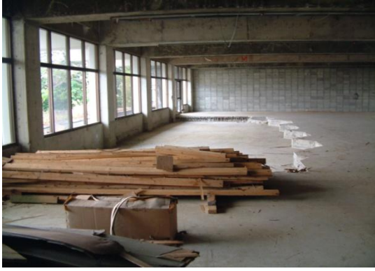
Restaurant on the first basement level
