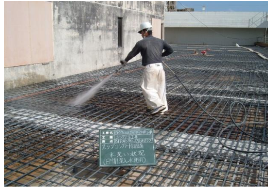
2. Application to reinforcing bars and forms
