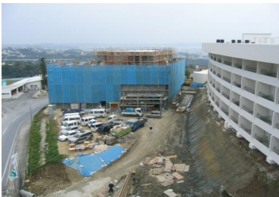
In Jan. 2006 Spa building under construction
