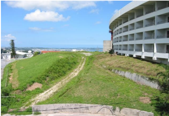
In 2004 before the repair work
